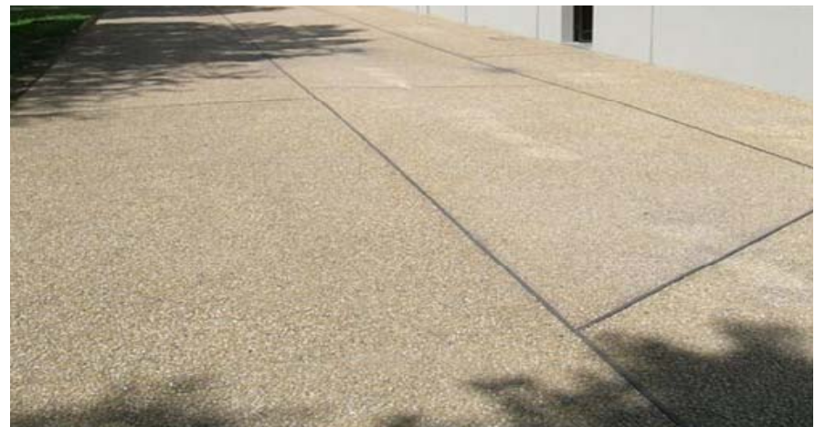
Exposed aggregate concrete to mark pedestrian crossings
